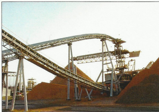
Chip piles and conveyors
