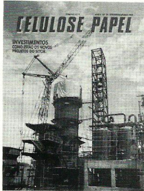
Cover: photo Klabin's Kamyr digester, under construction.
